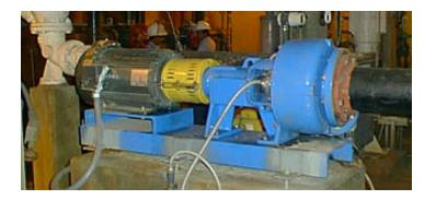
Discflo pumps are cutting energy and maintenance costs at US Filter's Wastewater Treatment Plant in San Diego County. Vertical dry pit Disc Pumps have replaced progressive cavity pumps at the belt filter press sludge feed station - one of the toughest applications at the plant.
