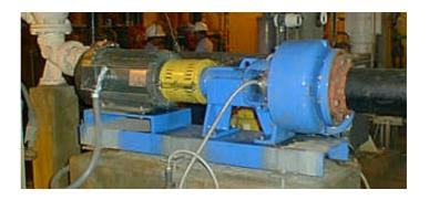
Discflo pumps are cutting energy and maintenance costs at US Filter's Wastewater Treatment Plant in San Diego County. Vertical dry pit Disc Pumps have replaced progressive cavity pumps at the belt filter press sludge feed station - one of the toughest applications at the plant.
